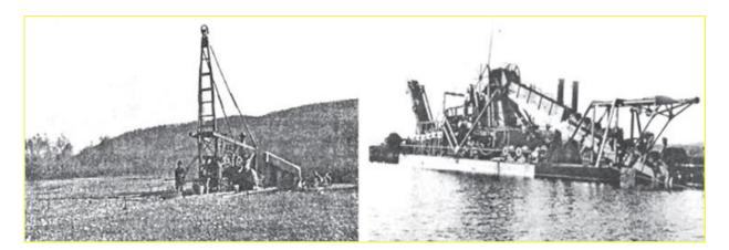
Exploratory drilling In the vicinity of Bor and mechanized excavation of gold-bearing sediments In the river Pek by a bucket excavator, early XX century
